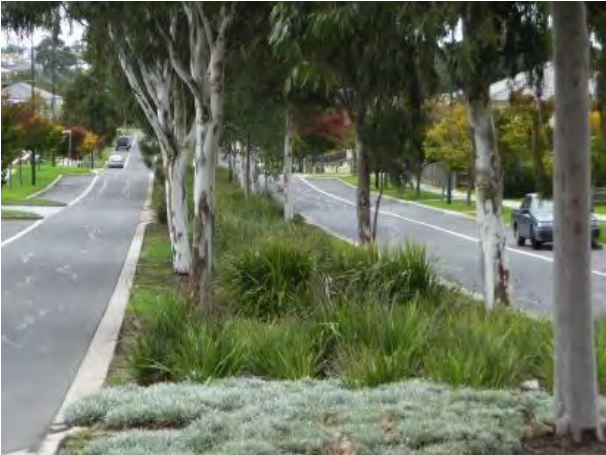
Drainage swales within road reserves (Class G Grassland)
