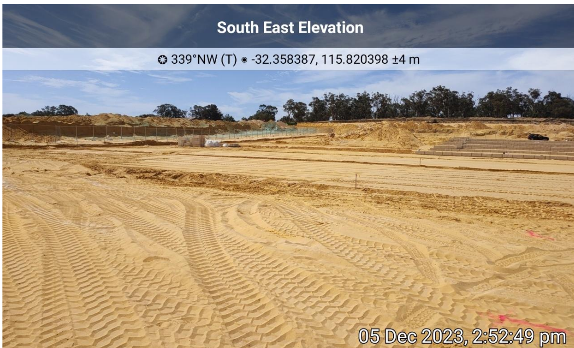
Plate 2: Evidence of site internals being cleared and maintained to low threat.
