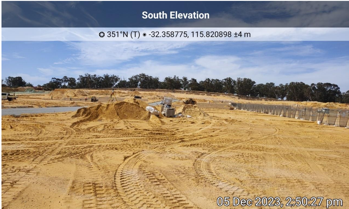
Plate 1: Evidence of site internals being cleared and maintained to low threat.
